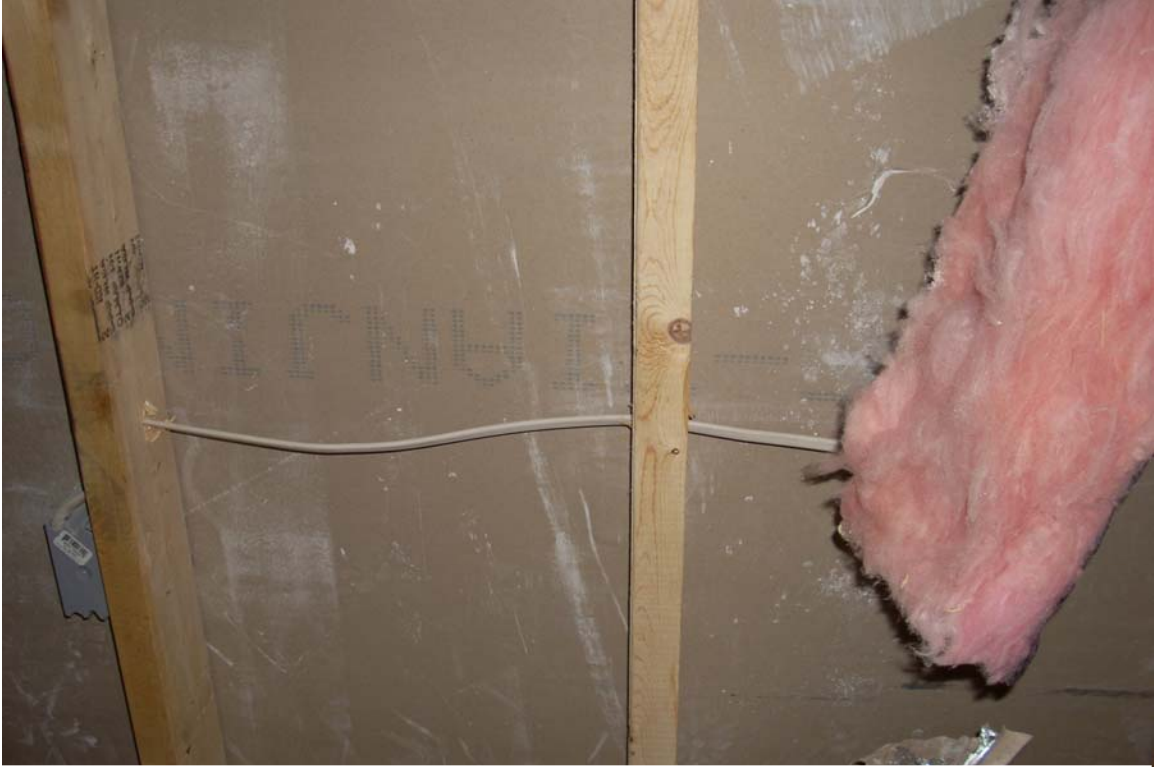
The backside of drywall may have a manufacturer's stamp making identification possible
